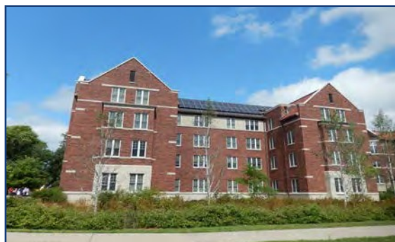
Rooftop Solar, CERTs
