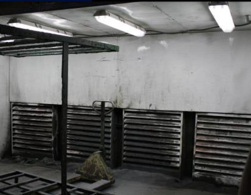
Paint booth after upgrade
