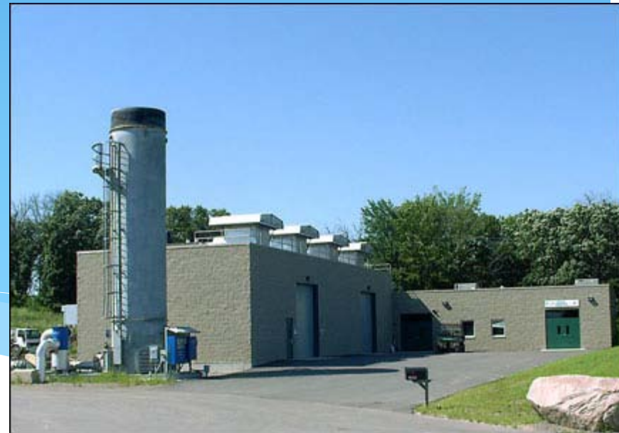
Above: Elk River's Landfill Gas-to-Electric Power Plant
