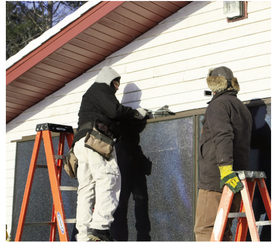
Solar thermal air heat panels being installed
