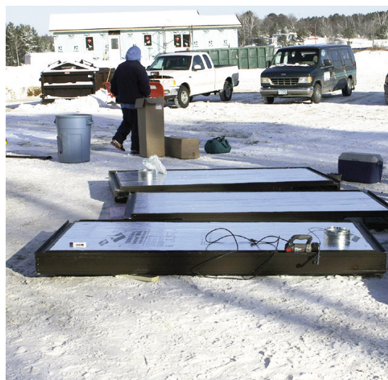
Solar thermal hot air panels ready for installation
