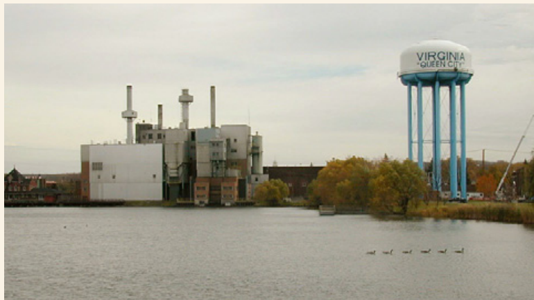
Virginia District Heating facility
