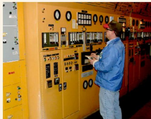
*Digester controls at a wastewater treatment plant*
