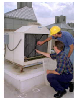
Cooling system inspection
