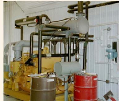
*Digester engine with heat recovery system*
