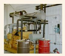
Digester engine with heat recovery system
