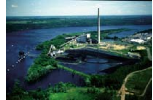
Large Electric Power Generating Plants
