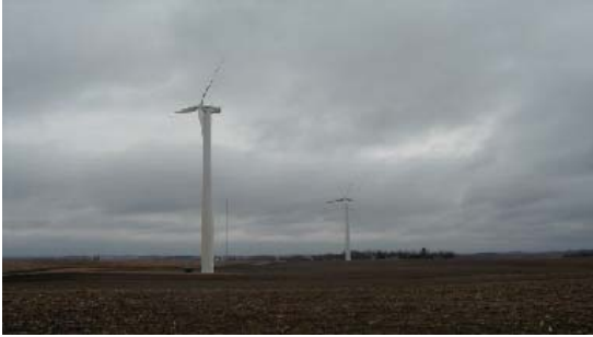
Large Wind Energy Conversion Systems
