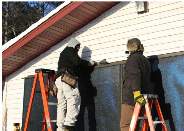
Installing a solar air heating system in northern MN
