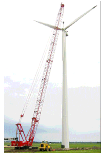
Construction of the Worthington wind turbine
