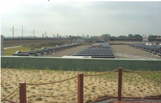
The green rooftop shares the roof with the solar panels
