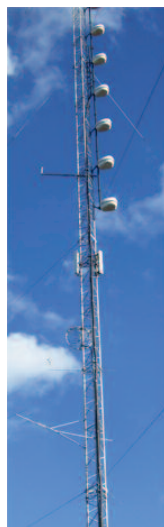
Lutsen communications tower with wind monitoring equipment
