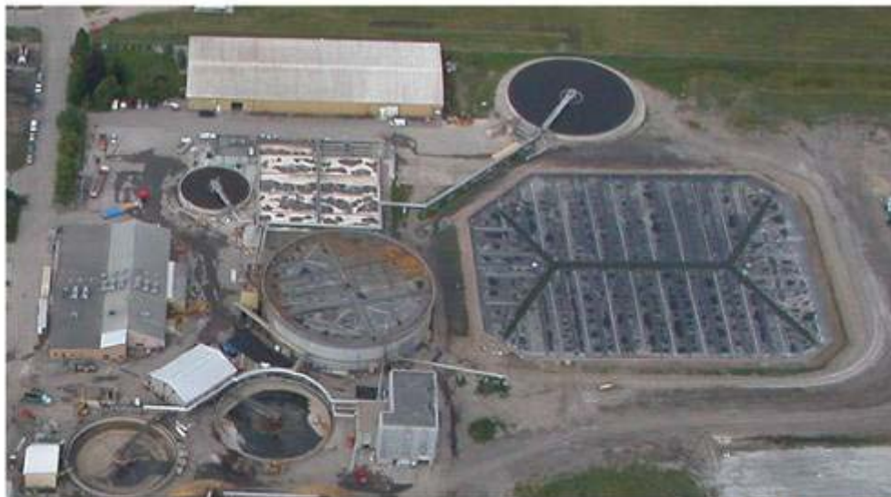
Figure 6 - American Crystal Sugar Company East Grand Forks Facility. Photo courtesy of American Crystal Sugar Company.
