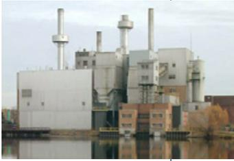
*By using waste heat, CHP can realize system efficiencies as high as 80%, nearly three times the efficiency of a typical coal power plant.*
