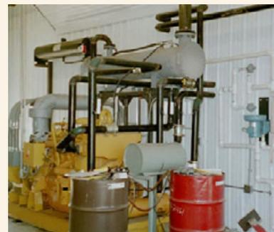
*Digester engine with heat recovery system*
