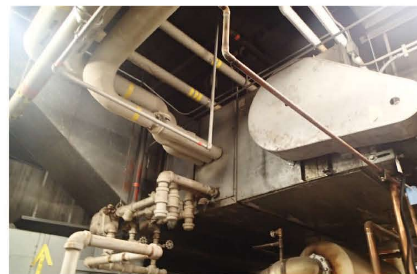
Corridor Ventilation Retrofit
