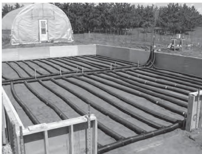
Figure 1. The lowest layer of tile line with the traditional high tunnel in the background.
