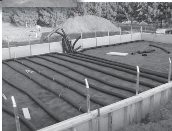
Figure 2. The second layer of tile line. The tile line was hooked up to the solar panels in the center of the picture.
