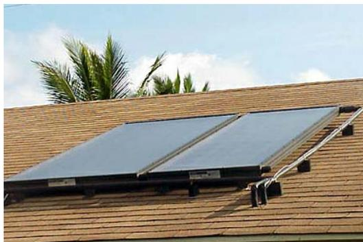
*Flush mounted solar hot water panels*
